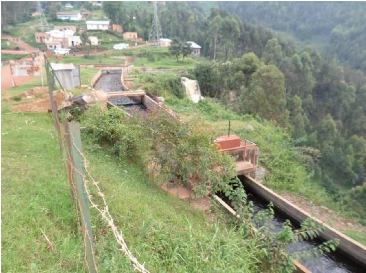
Photo 6: Hydropower station constructed on Rugezi falls
